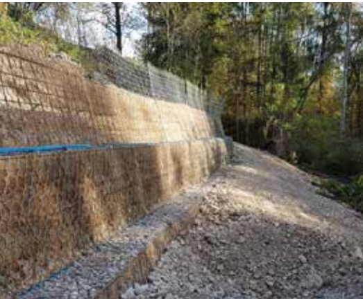
Einbau bewehrte Erde, System Green Terramesh, Fa. Beco Bermüller
